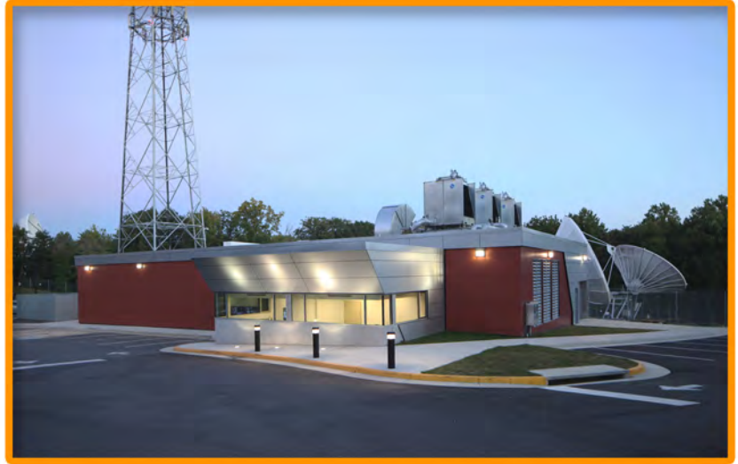
PBS Technology Center; at right are the "Ku" west and "receive only" dishes; at left is the microwave tower supporting the feed to/from PBS headquarters
